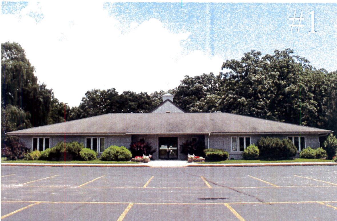
#1: Front of Building Front Faces West Camera Facing East Taken 7/8/14 At 12:15pm
